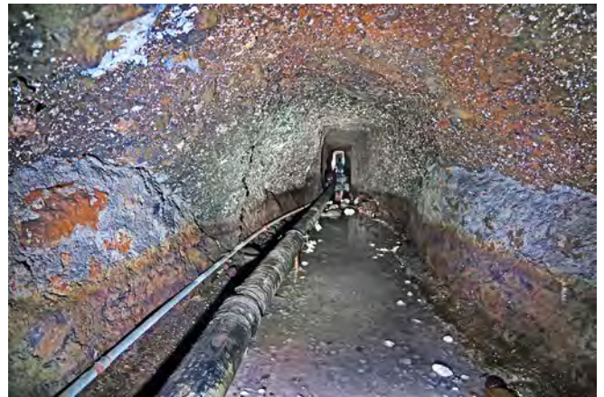
In places the amount of water seeping through created pools a foot deep. Calcification leaving white deposits everywhere and some splendid 'cave pearls'.
